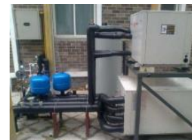
Ground source heat pump
